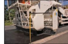
A metered spreader puts hard stone chippings on to the hot bitumen.
