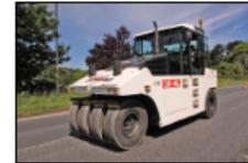
These chippings are then lightly rolled and pressed into the bitumen to form an interlocking surface.
