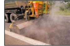
A calibrated tanker sprays a thin film of hot bitumen on to the road.
