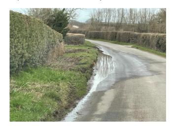
**Sinton Green, vicinity of the The Forge -** Water suggested to be originating from garden water feature; water in road; sodden, damaged, eroded verge; overgrown hedge.
