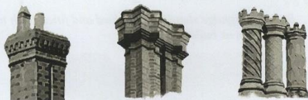
Examples of ornate chimneys
