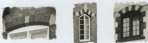
Examples of variations in detail between buildings
