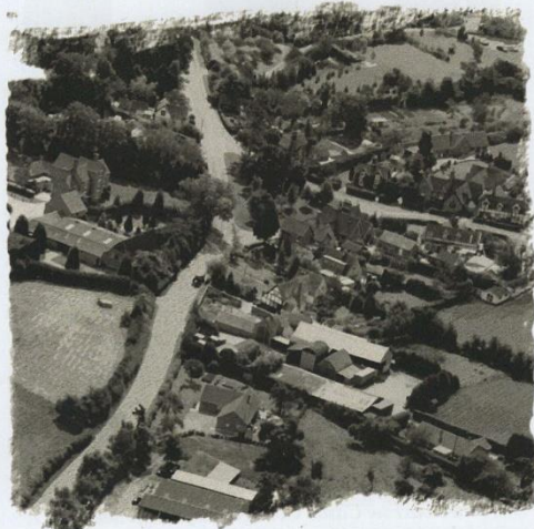
An aerial view of the settlement around Rous Lench village green
