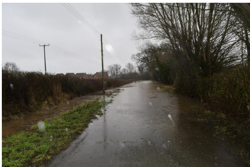
Floods on Link End Road near Poolhay January 2021
