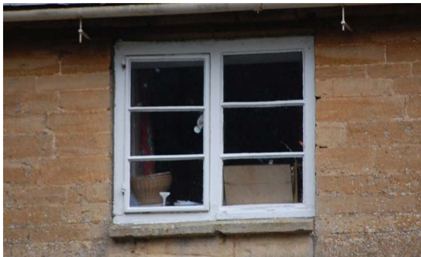
Figure 10. A typical, three-pane, iron casement window.
