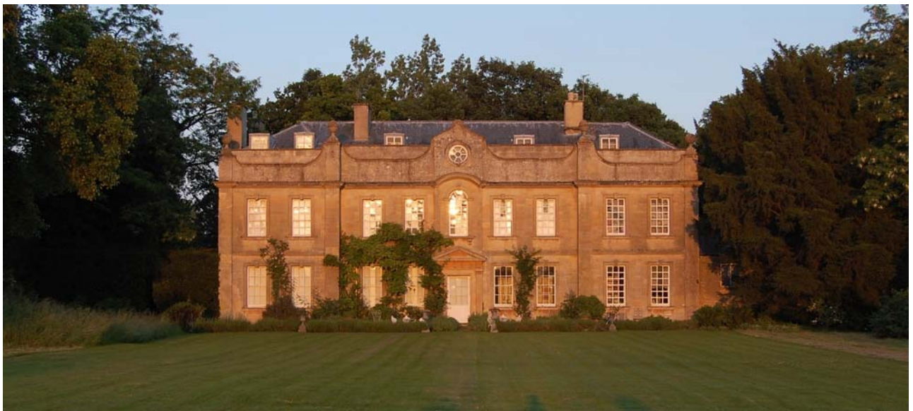
Figure 9. West façade of Kemerton Court, built from local limestone ashlar, c. 1720.
