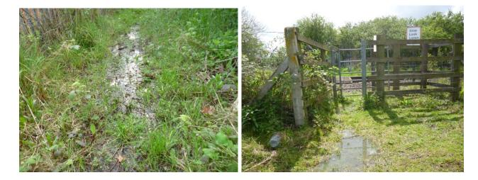
FIGURES 6.3-6.4: Waterlogged conditions on footpath and railway crossing adjacent to path
