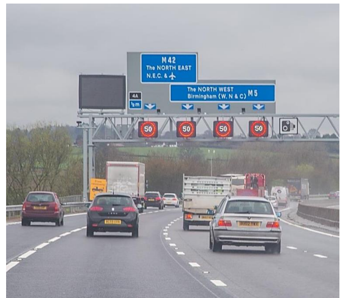
Signs and signals being tested on the M5 between junctions 4a and 5
