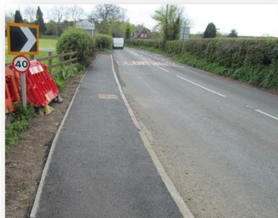
Hackmans Gate Lane new footway
