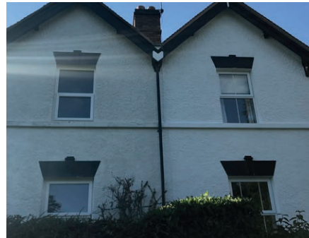
Examples of poor uPVC replacement windows (Upper and Lower Wyche)
