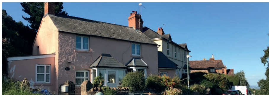
Example of extensions (right and left) to an historic house that do not match the pitch or material of the original roof, use windows of a different proportion and materials that copy, rather than complement, the original building (RCA06 Upper and Lower Wyche)
