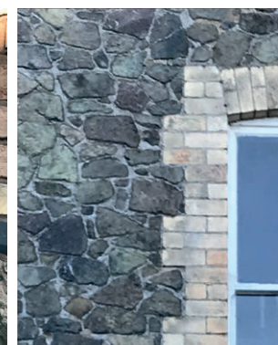
Malvern Stone used with buff engineering bricks
