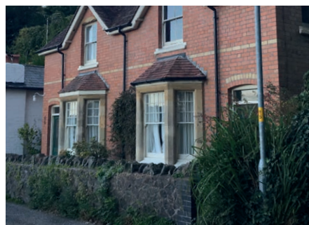
'Cock and hen' coping on traditional Malvern stone wall, Holywell Road
