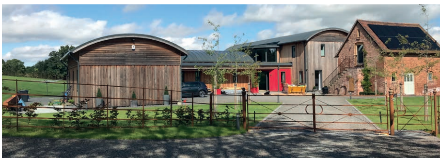
Farmstead conversion does not reflect traditional form or materials, using curved roofs in reflective material and timber boarding (LLCA08 Mere Brook and LNR)
