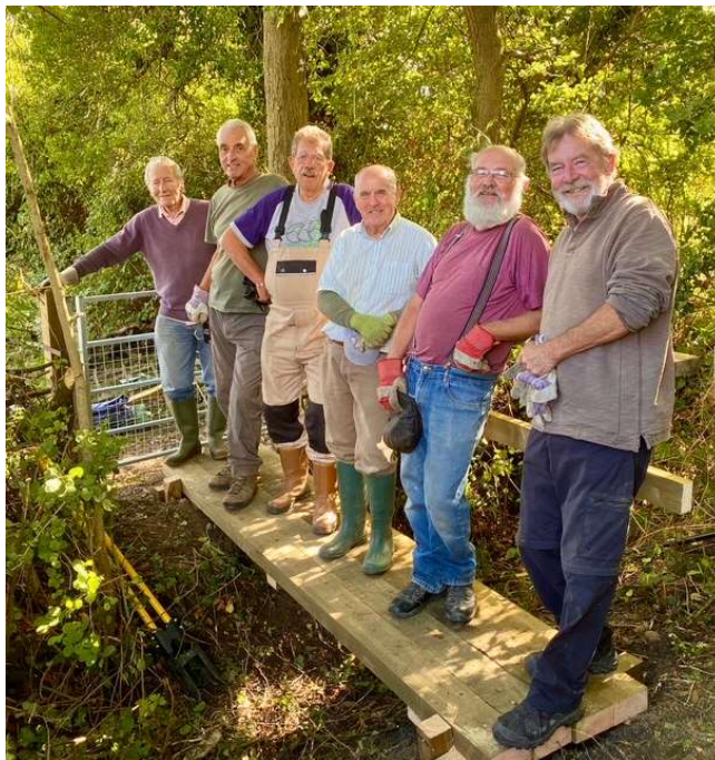
New Gate & Ditch Crossing Installation – 'The Slinget'
